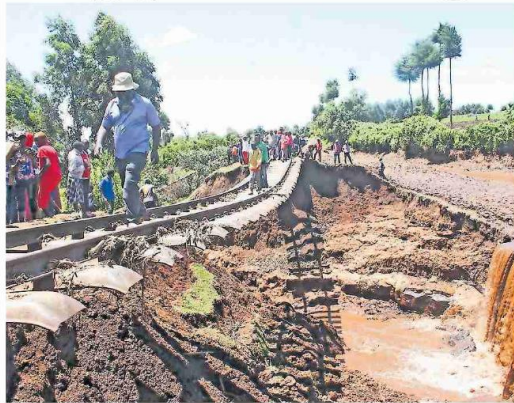
Oblivious of the danger they face, pedestrians use a suspended railway track after flood waters washed away the soil and caused gully erosion in Elburgon, Nakuru County, yesterday, following a heavy down pour. Farms were destroyed and trees washed away.
